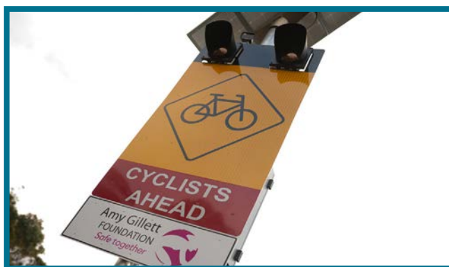
Dynamic flashing warning lights (Victoria)
