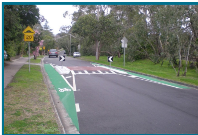
One-way slow point with bicycle-bypass facilities
