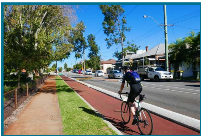
Bike lane protected with concrete kerb
